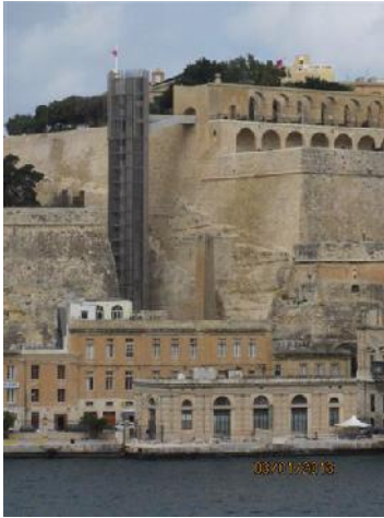
The new Baracca lift
